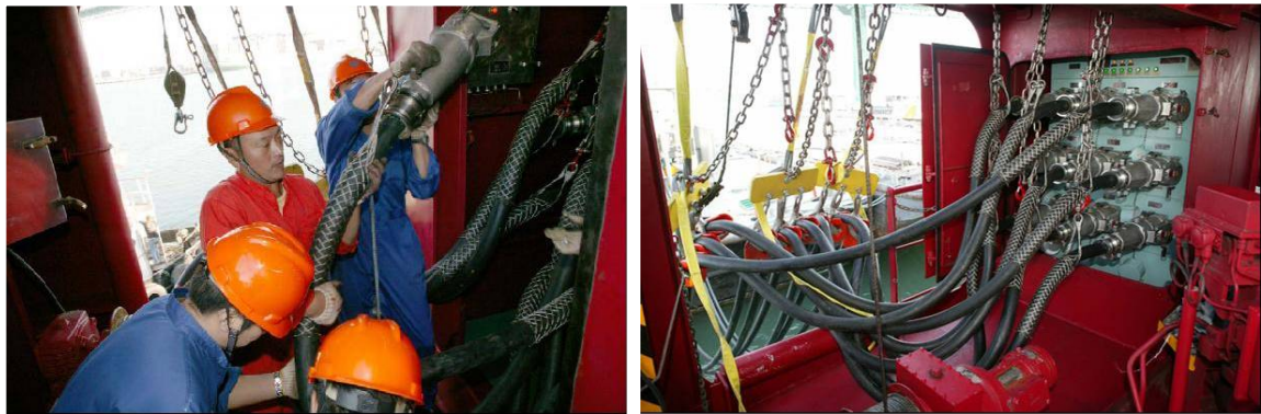
Figure 14 Installing a 440 V connection on board
